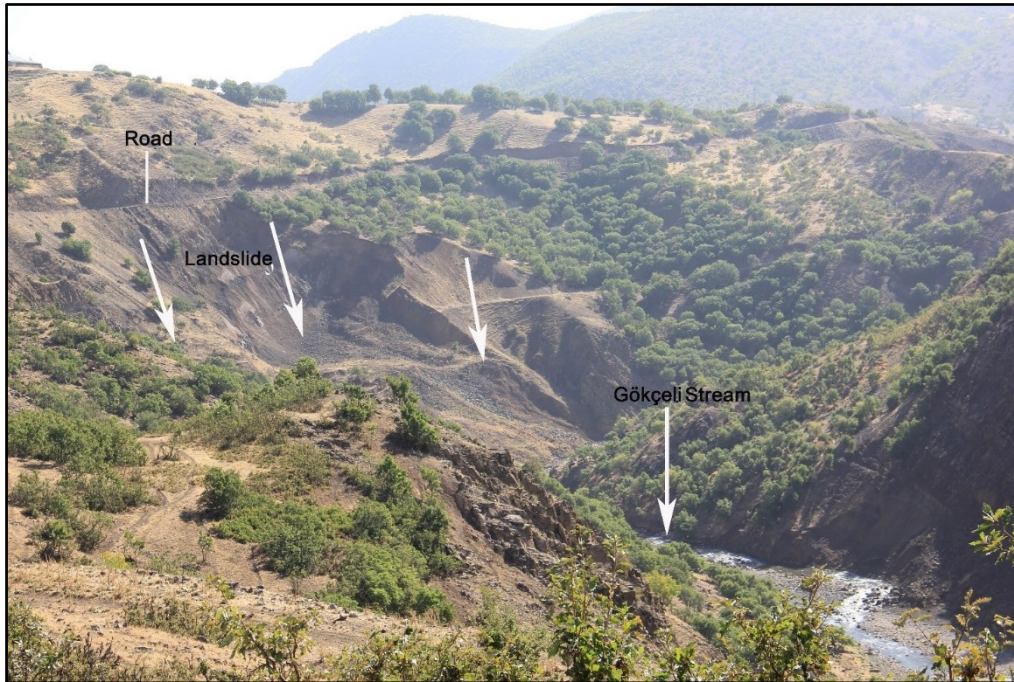
Photo 3. Erbaşlar-Adaklı Highway is affected by landslides.
