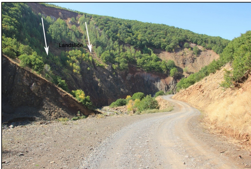
Photo 5. In Adaklı, landslides have occurred in areas with heavy vegetation as well.
