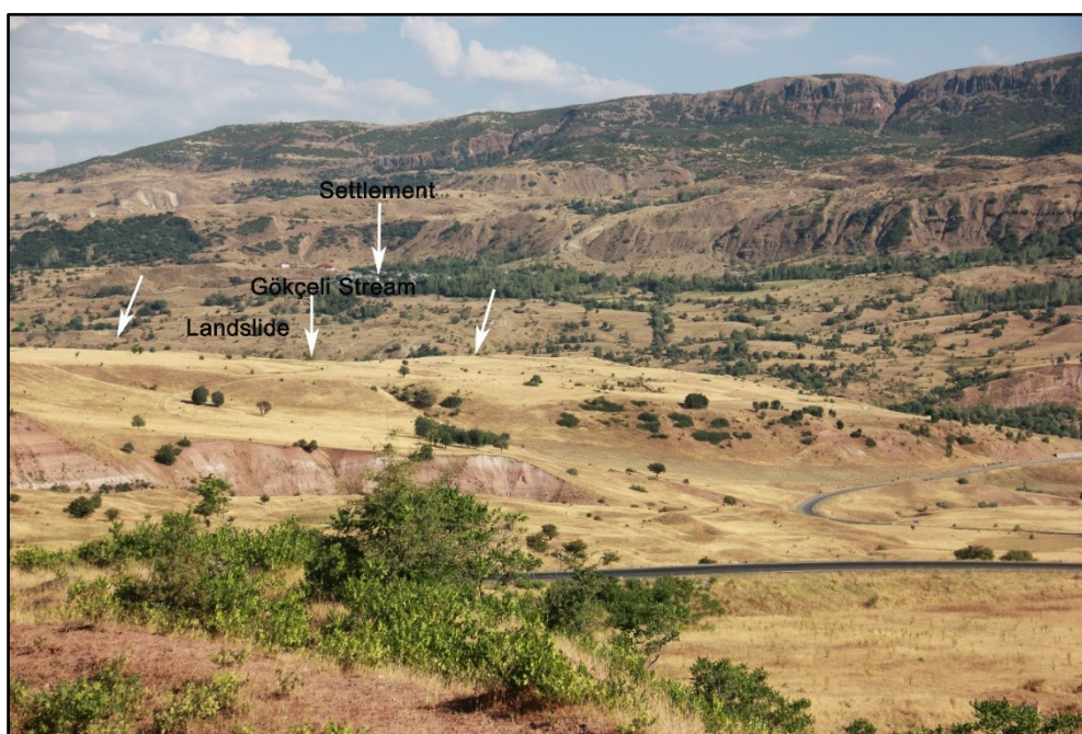
Photo 4. Settlements on the hillsides of valley in Gökçeli village are affected by landslides
